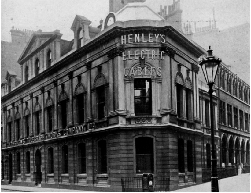
Henley's electric cables
